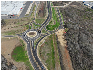
The new turbo roundabout (2nd in the country) outside the new J.M. Smucker facility in McCalla.
